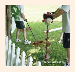
Each year, we identify and investigate unauthorized activities (UAs) that occur close to our pipeline right-of-way. A UA is an activity that contravenes the Canada Energy Regulator (CER) safe digging regulations or that doesn't meet Trans Mountain's requirements for working safely near the pipeline. One of the most common causes for a UA is a ground disturbance carried out by a property owner or contractor without placing a locate request with a local one call service.
