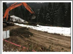
Forest debris used for topsoil cover as an erosion control measure.
