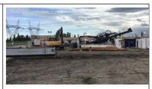
Directionally drilling a small diameter pilot hole.
