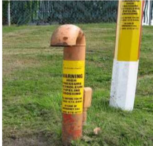
Casing Vent Marker
