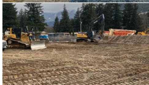
Images of topsoil stripping at Road 59.
