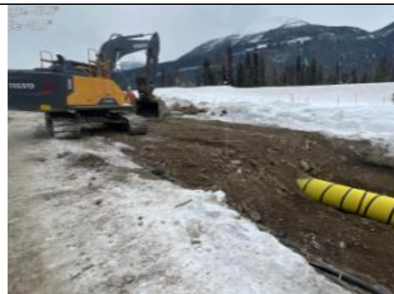
Backfill in progress at KP 433.
