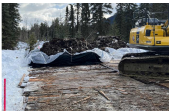
Wetland topsoil stored separately from upland soils at Dig 42 KP 432.
