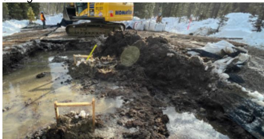
Topsoil stripping at Dig 42 KP 432.
