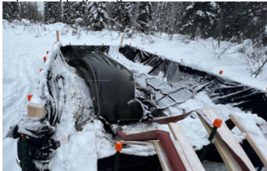
Sediment trap in use for pump-off at Dig 46 KP 432.
