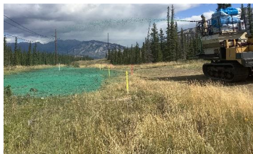
Hydroseeding equipment in use.
