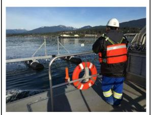
Indigenous Monitor inspecting bird deterrents on the marine construction safety boom. The Canada Energy Regulator also inspected the deterrents during a regulatory inspection and asked the Indigenous Monitor questions about the effectiveness of these deterrents.
