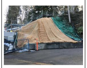
Coco matting and hydroseed (green) installed on steep slope for erosion and sediment control.
