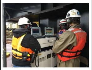
Environmental monitors and Contractor Superintendent monitoring underwater noise levels during offshore impact pile driving.
