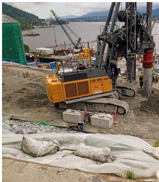
Secant wall construction at WMT.
