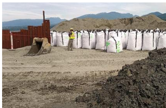
Super sacs filled with gravel ready to be placed in wall.
