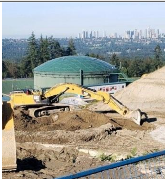
Contaminated soil excavation at Burnaby Terminal.
