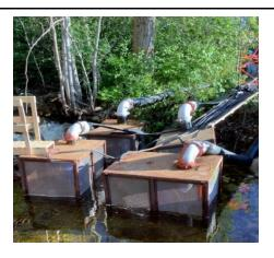
Upstream diversion pumps used in conjunction with an Aqua Dam isolation to successfully divert and maintain watercourse flow
