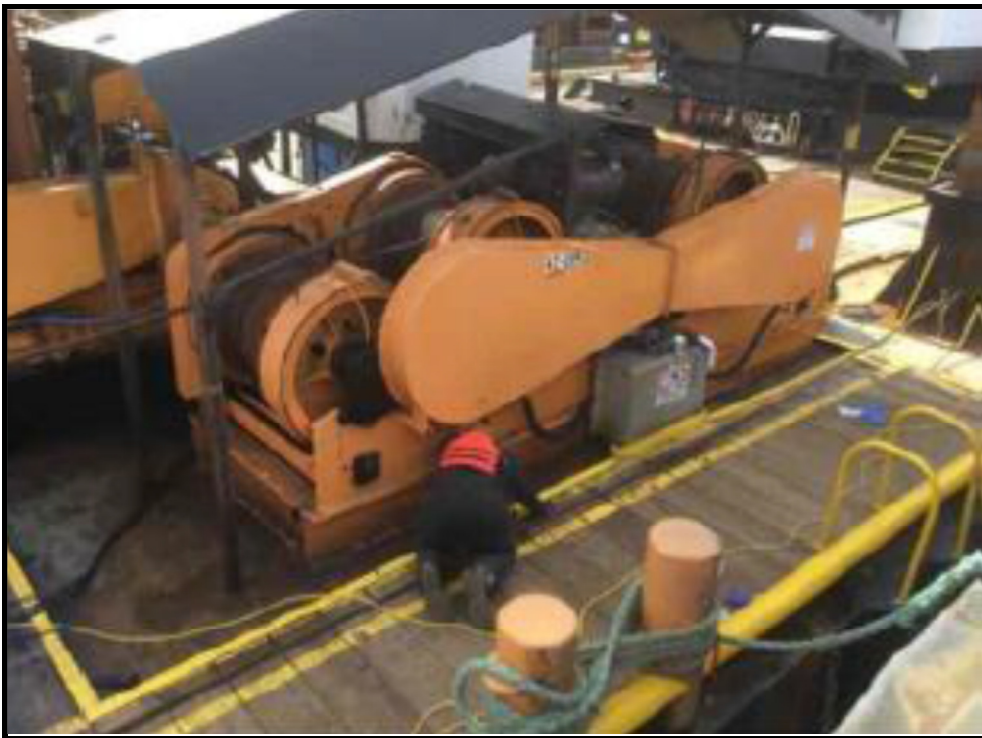
Photo 002_20180503: Crew installing secondary containment around deck winch on DB Olympia.
