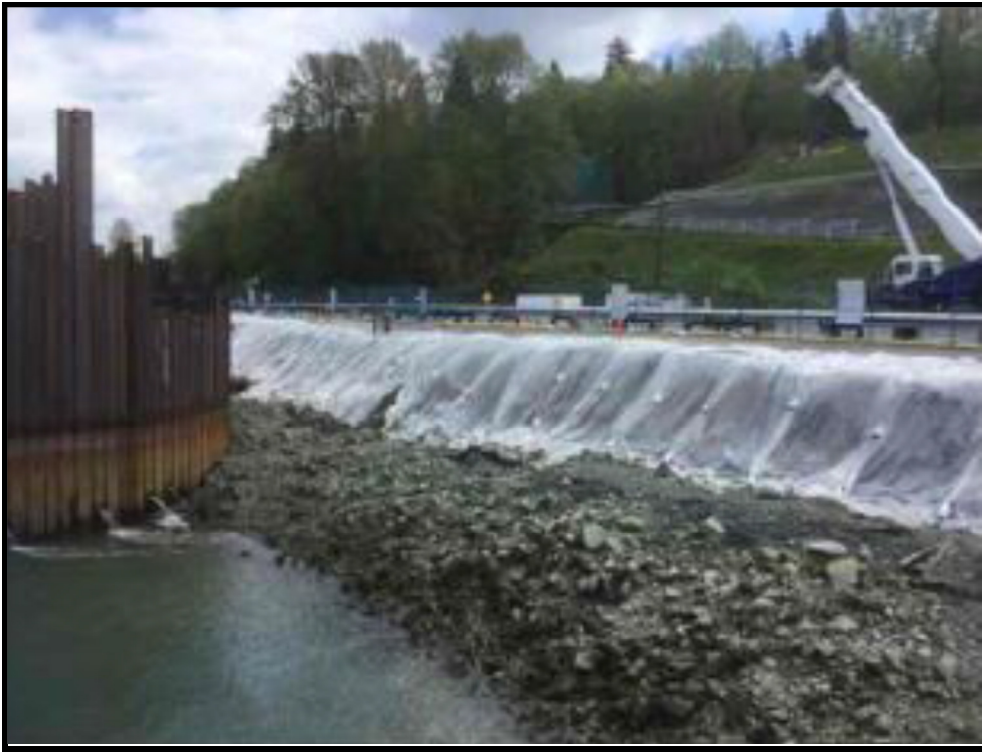
Photo 002_20180501: Poly sheeting installed along shoreline to protect backshore sediment.
