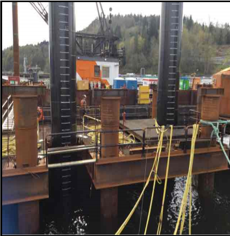
Photo 004_20180418: Crew installing bubble curtains around Piles J and K.
