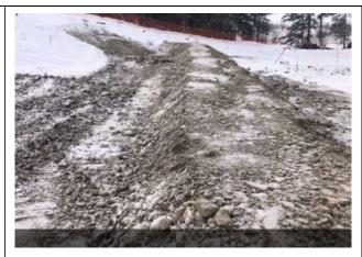
Diversion berms to displace water away from right-of-way.
